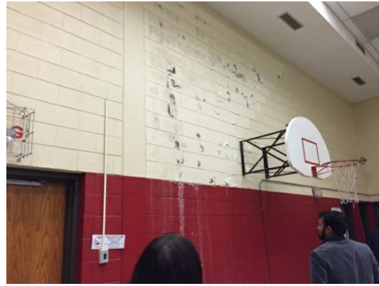
Interior damage from roof leak
