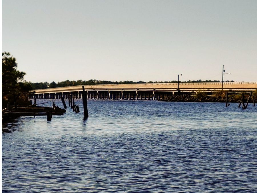
Figure 7 Boat Launch at Roper Ditch Source: Michael Cole
