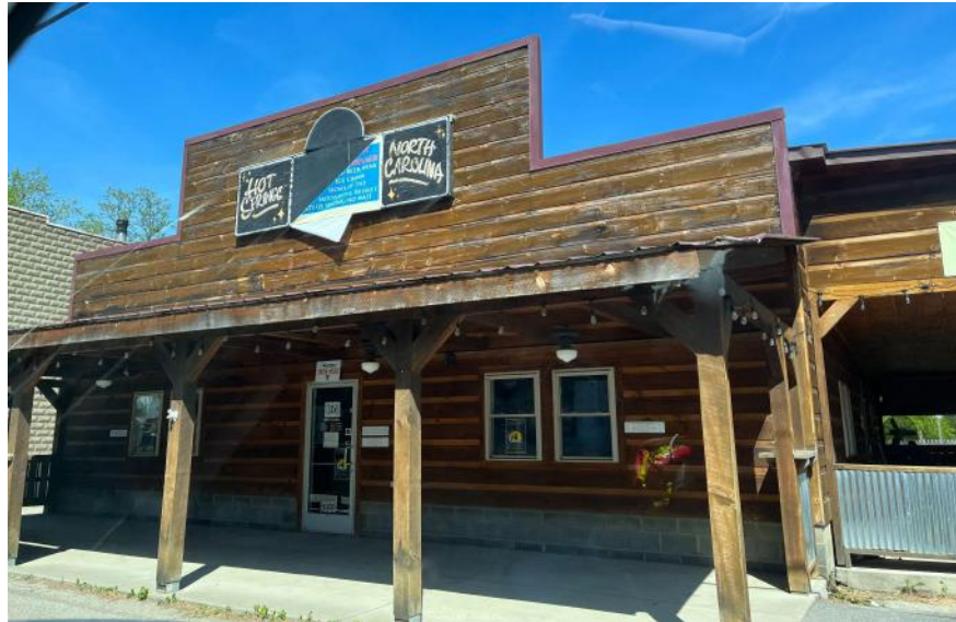
Workshop participants cited renovation of aging and distressed structure as important for staying connected to the town's history
