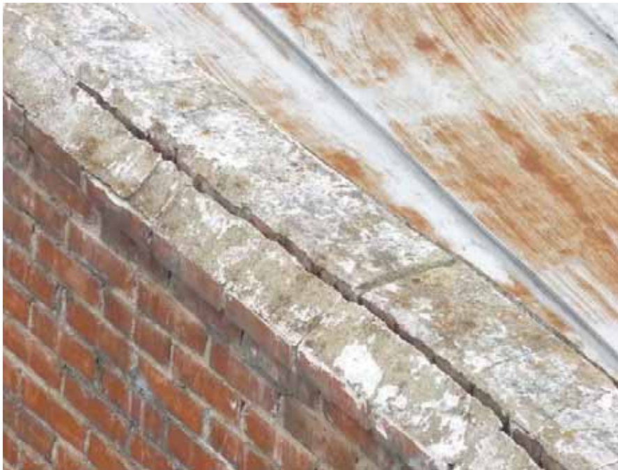
112. Building T - parapet cap is in need of repair.
