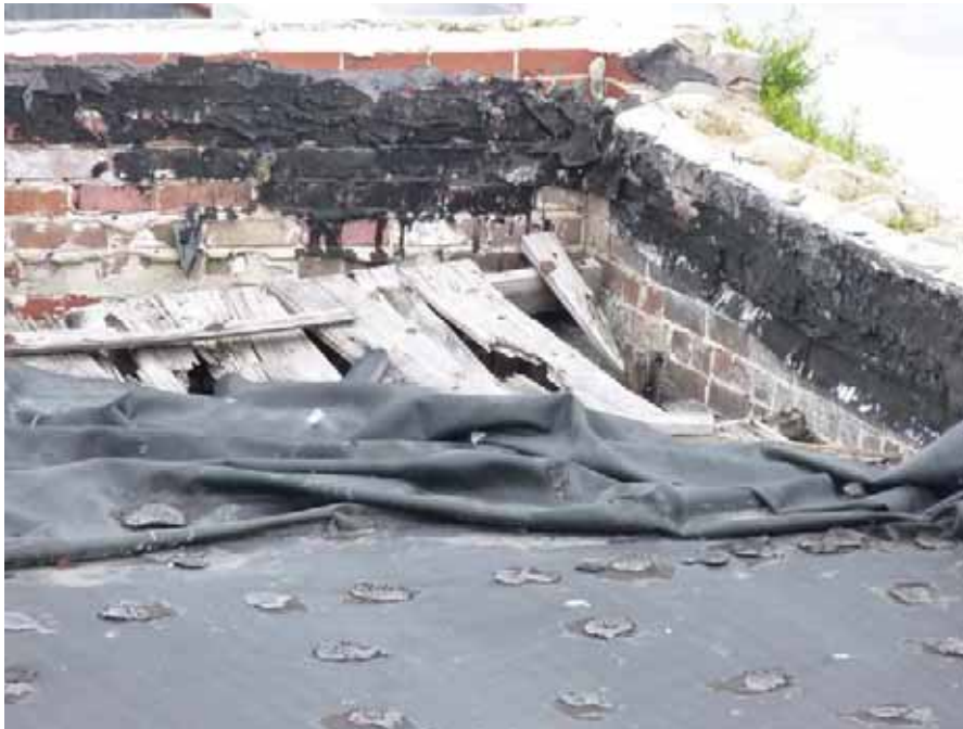
104. Building S - closer view of deteriorated wooden roof deck.
