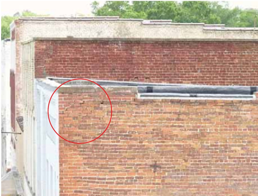
40. Building I - Parapet needs repair.I
