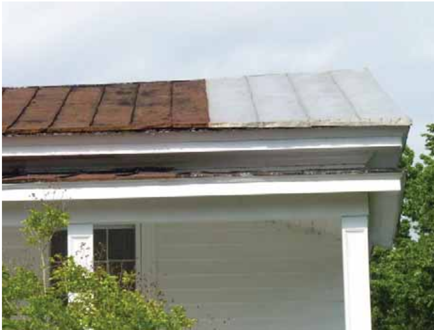
137. Building X - some metal panels have been coated.
