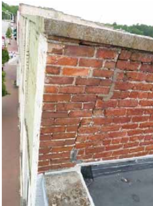
44. Building J - Parapet needs repair.
