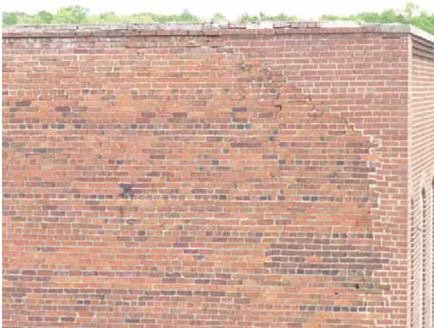
93. Building R - previous masonry repairs.
