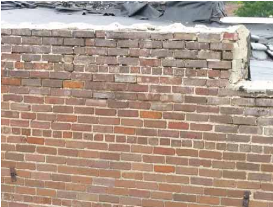
106. Building S - parapet repair is needed here.
