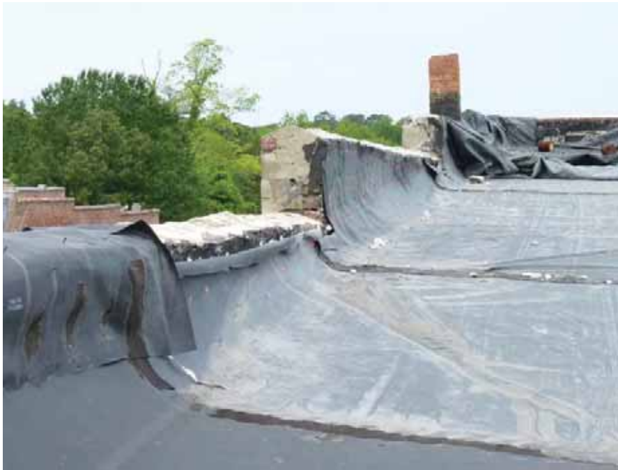
101. Building S - water may enter at the parapet flashings.
