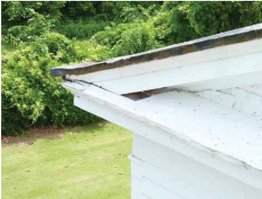
139. Building X - water table flashing does not extend fully across the top of the water table; water may enter here.
