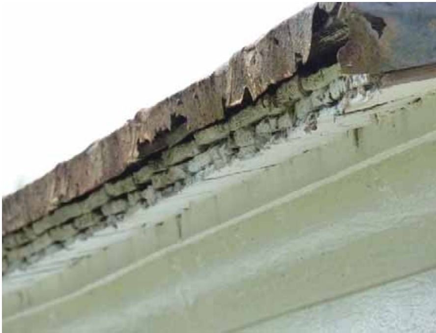
144. Building X - metal panels have been installed over the original wood shingles. Metal is severely rusted at the eave.
