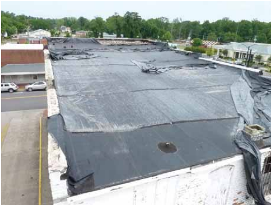
100. Building S -rubber sheets have been applied in an attempt to protect the building, however, many sheets have been displaced by wind forces.
