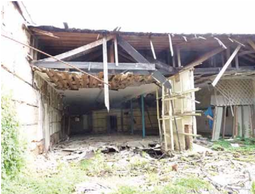
78. Building Q - rear 20' of the roof structure has collapsed; note the charred roof truss members as evidence of fire damage.
