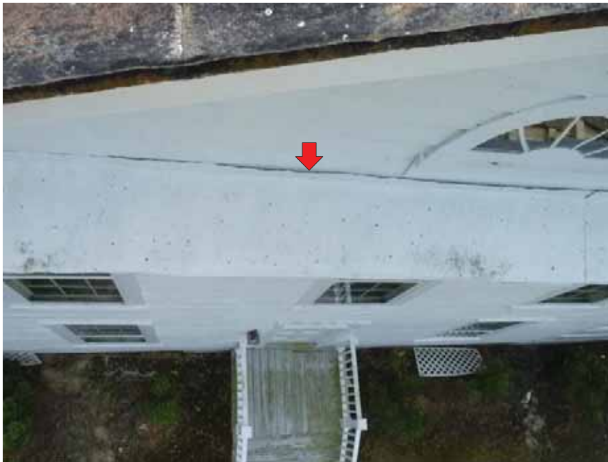
140. Building X - looking down on water table; sheet metal flashing is open at the top and water may enter here.
