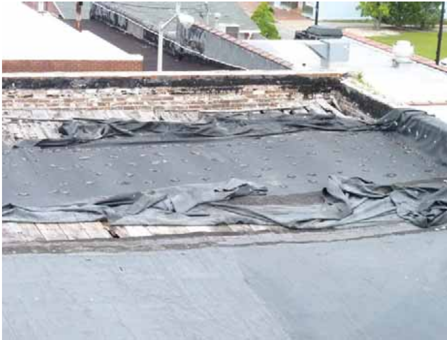
103. Building S - wooden roof deck is exposed to the weather at many locations.
