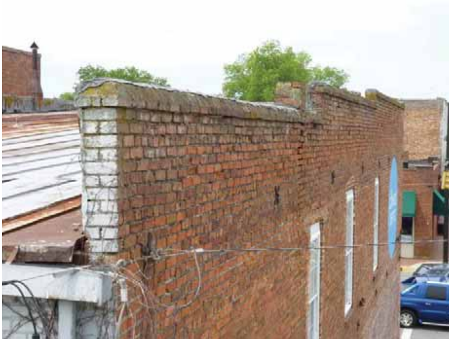
131. Building W - masonry repair needed here; see also next photograph.
