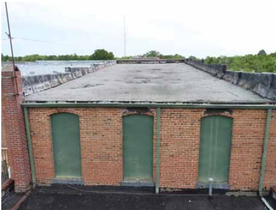
116. Building U - roof structure sags at the rear of this roof.
