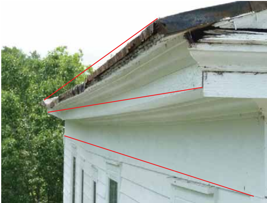
145. Building X - eave and wall sag; red lines have been added as a reference.
