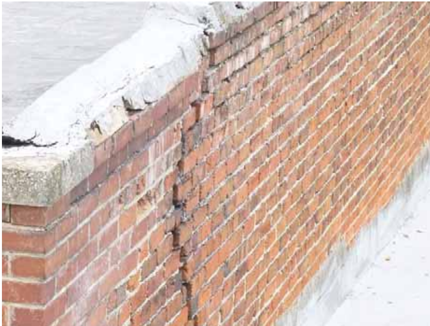
92. Building R - masonry repair is needed here; a similar condition may have existed at the opposite front corner as shown in photograph 93.
