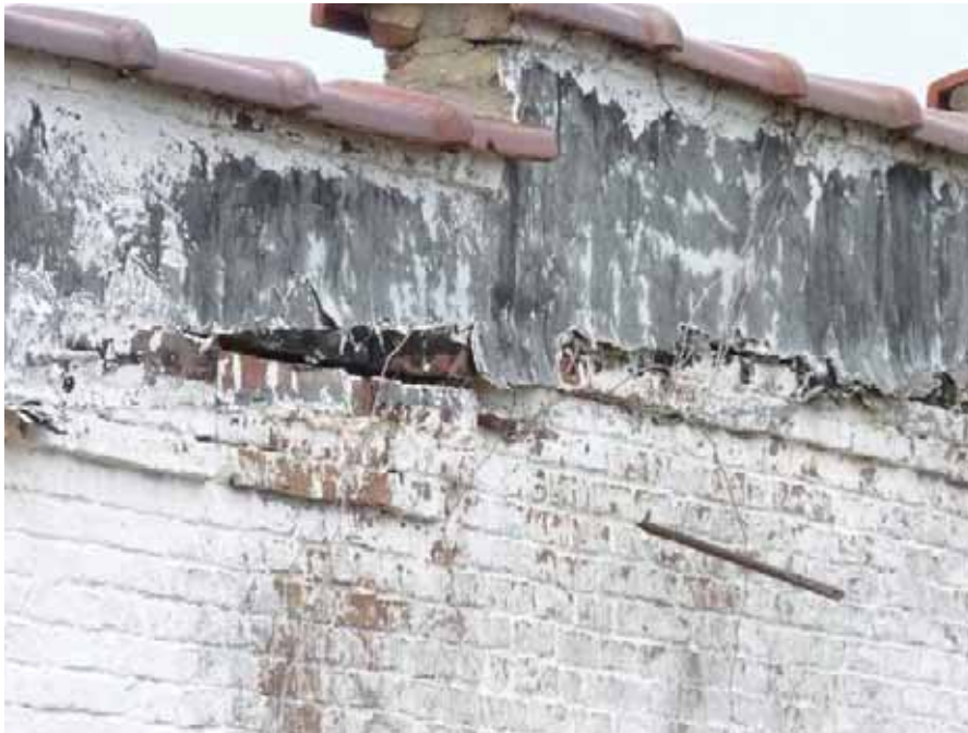
70. Building P - minor parapet repair is needed to fill the raggles where the counterflashing was removed.
