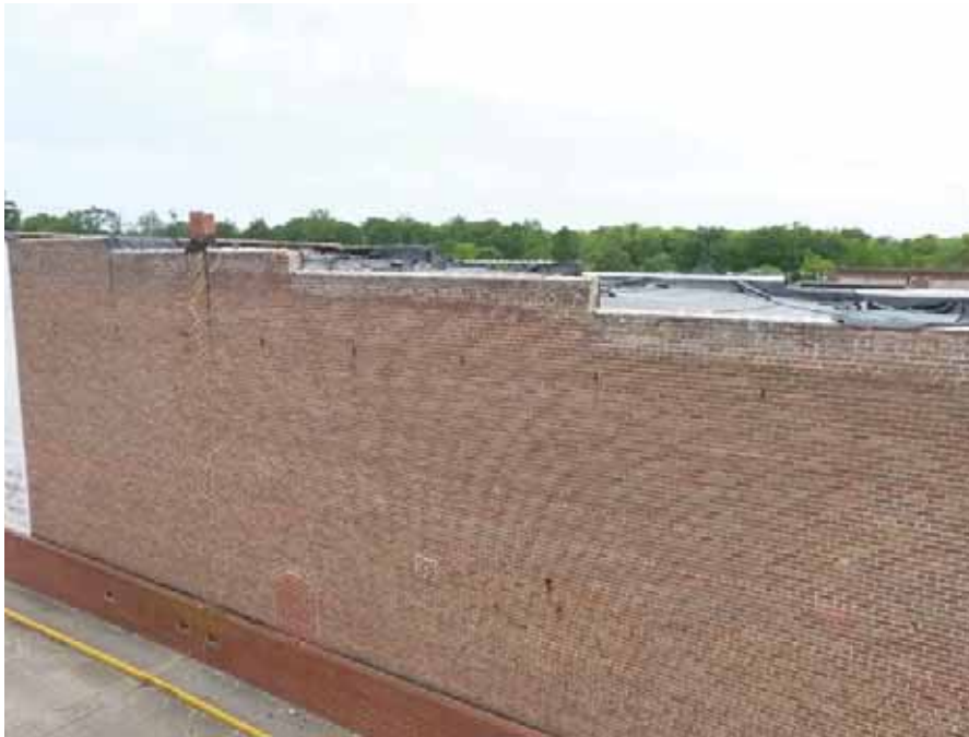
105. Building S - parapet repair is needed; see closer view in photograph 106.
