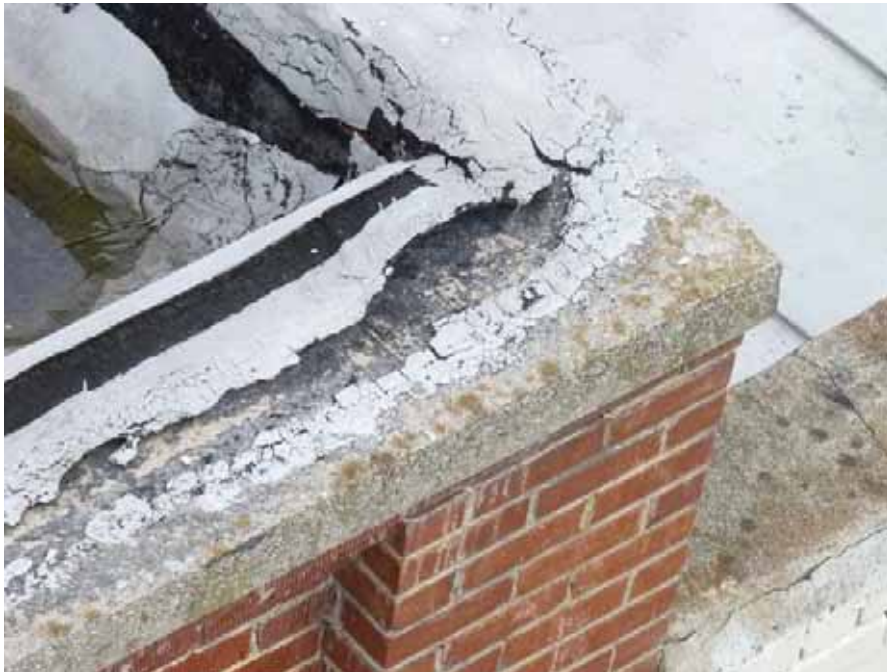
90. Building R -flashing at parapets is slipping and has pulled loose from the top of the coping.
