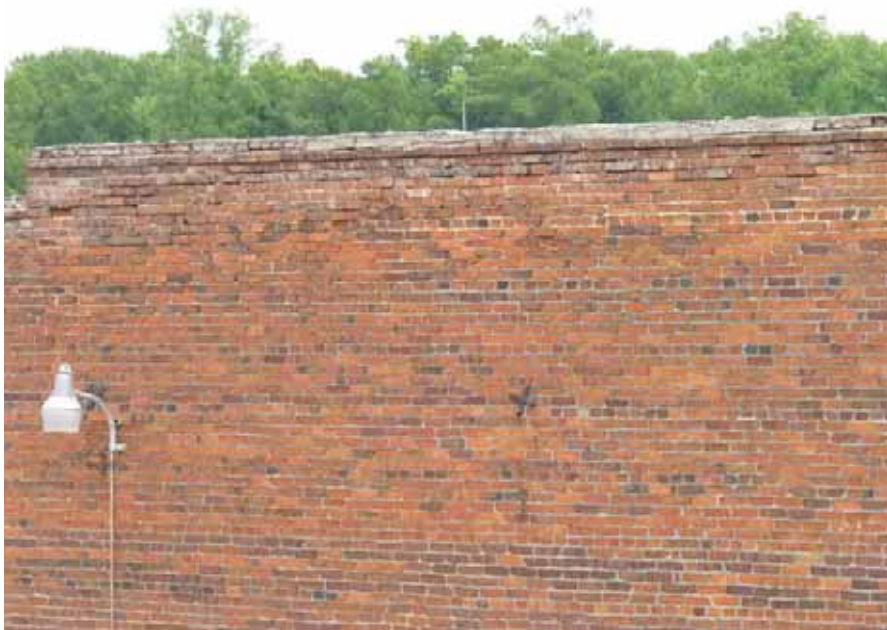
94. Building R - masonry at parapet needs repair; see closer view in photograph 95.
