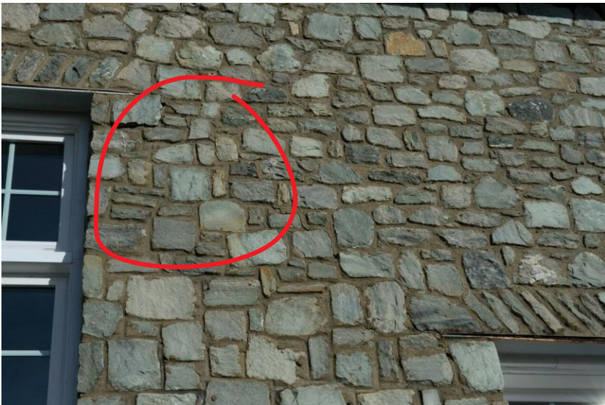
Pictured above and below: Cracks over windows.
