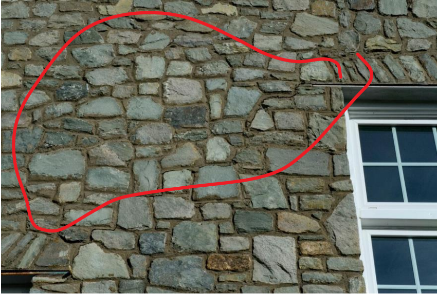
Pictured above and below: Cracks over windows.
