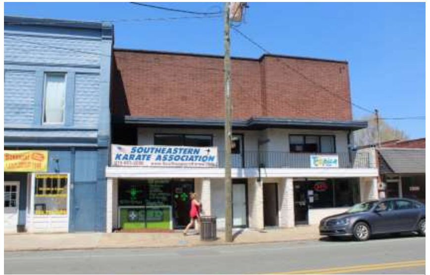
Figure 15: Street view of 112-118 W. Swannanoa Street which currently houses a variety of business: A CBD shop, tanning salon, and karate studio.
